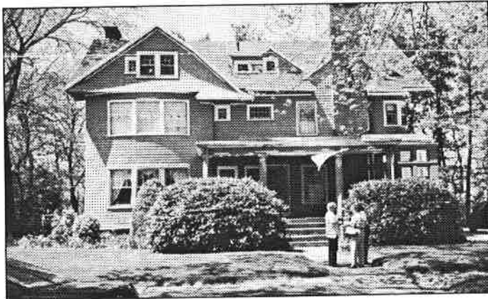
70 Bellevue Avenue has a restored greenhouse (lower right corner of house).
