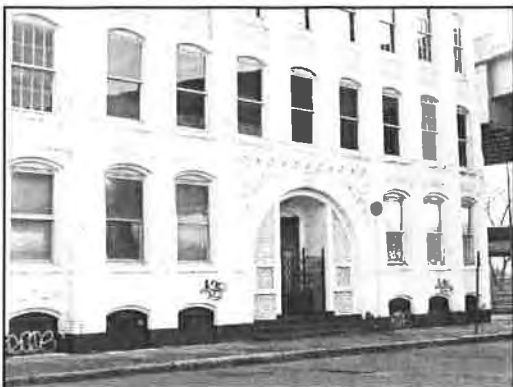
Kittredge Building, East Columbus Ave.
